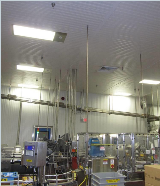
Walk able ceiling
