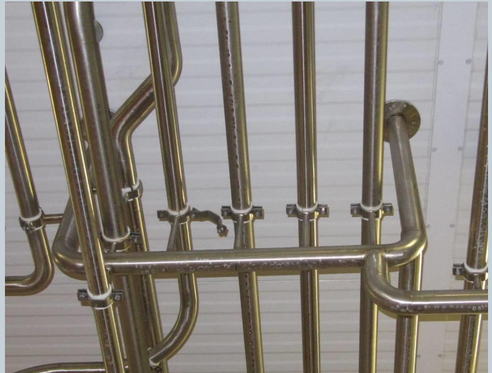
Sanitary process piping hangers and installation
